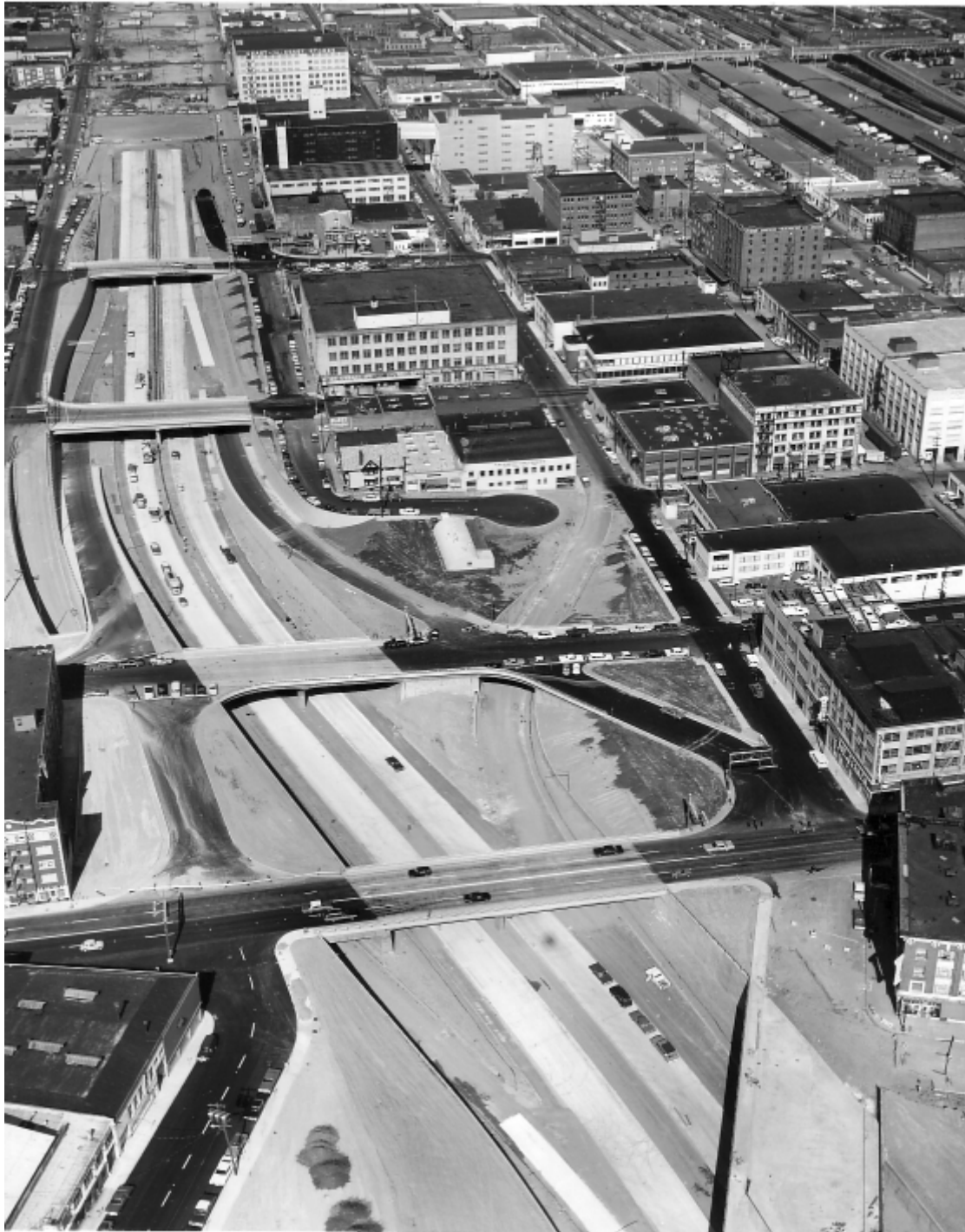
Figure 30. Interstate 405 “Stadium Freeway” construction, October 1968 (Source: ODOT GF, Image A362-9).
